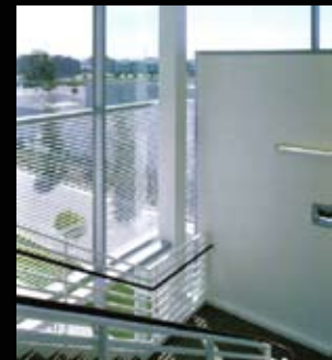
fig.20 Day light stairwell
