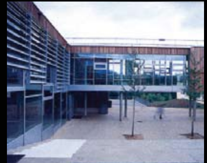
fig.25 Naturally lit transition spaces
