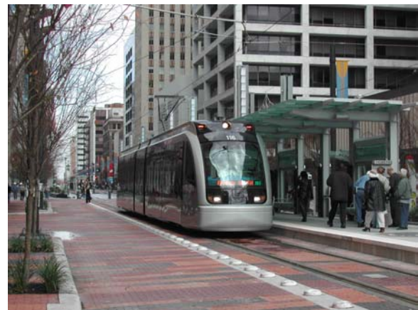
Figure 2.52 Light-rail Station, Houston Light Rail 11
